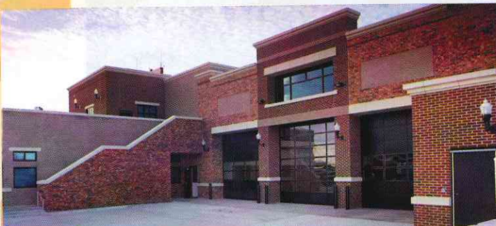
Hurst Fire Station #2
